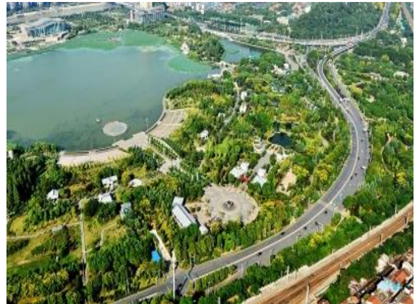
Six Lakes interconnection project in Hanyang
